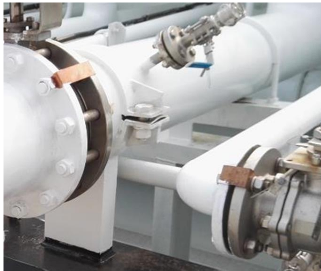
Figure 5.5.3.2 Pipe connection against static electricity
