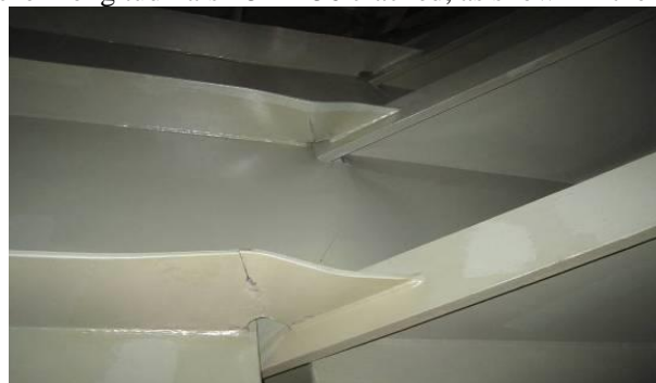
Figure 4.4.5.1(3) Deformation
